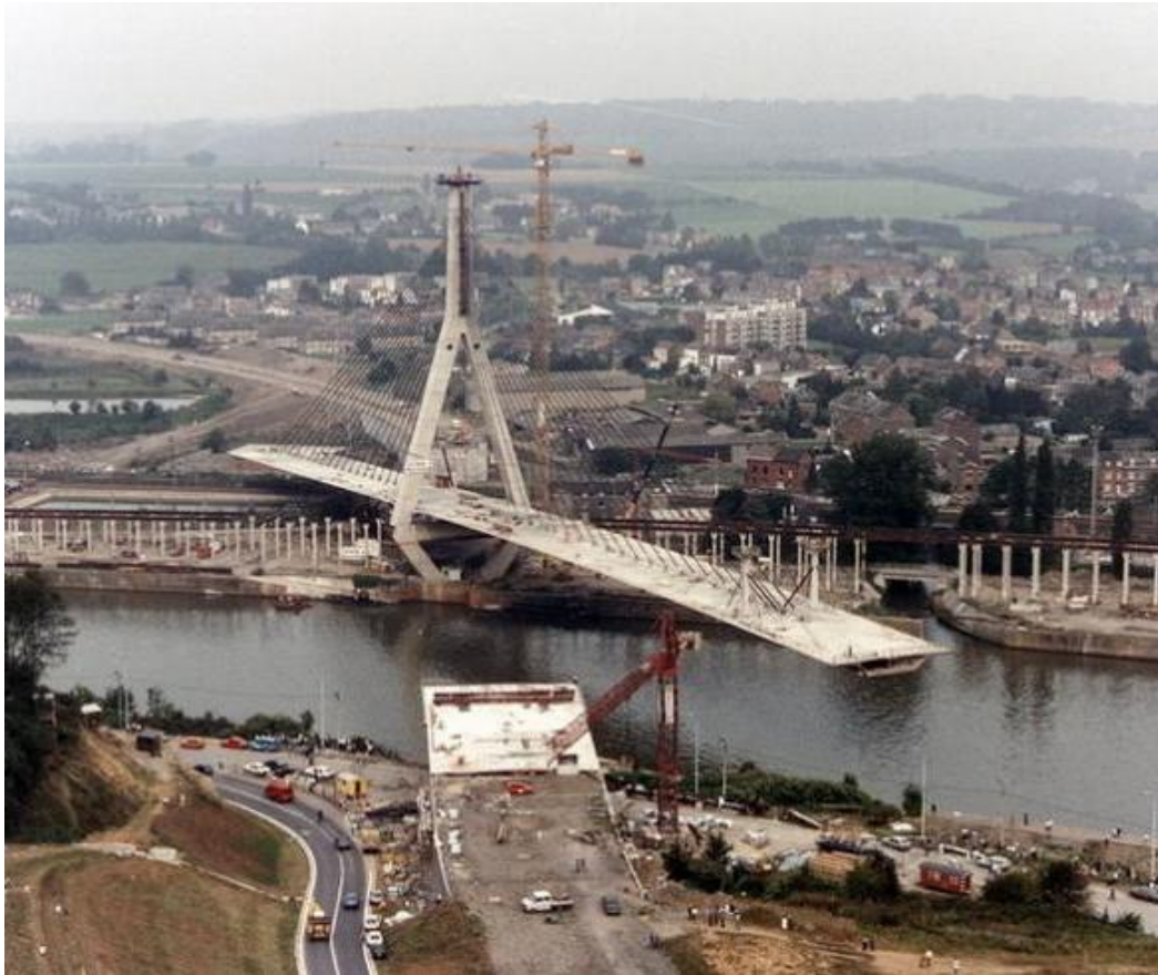
Figure 3.5. Cable stayed bridge installed by rotation in Huy, Belgium (Source: Duchene)
