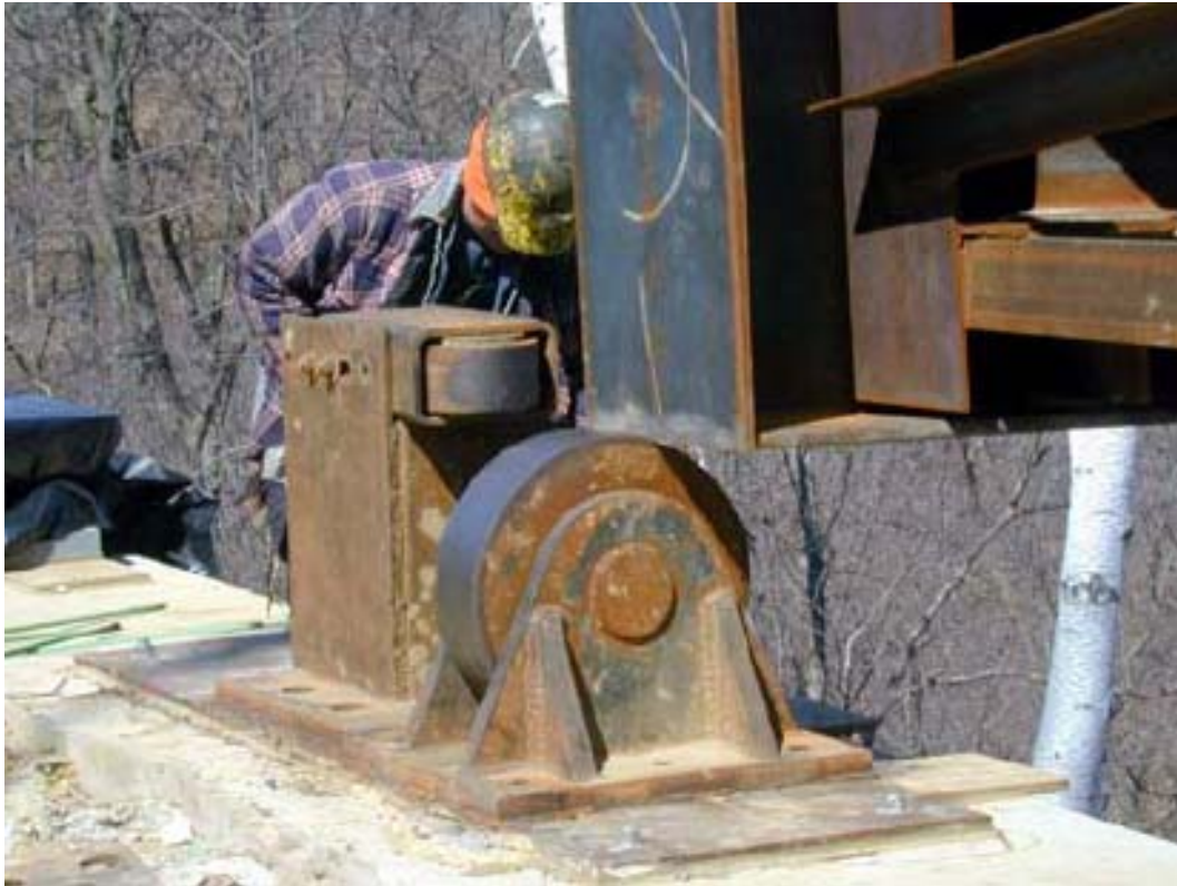
Figure 3.2. Temporary supports used during the launch to minimize the friction at the piers [4]
