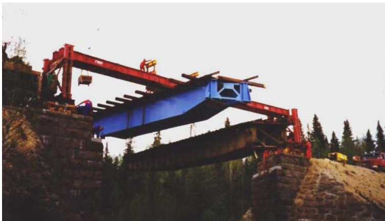
Figure 3.11. Bridge replacement by double rotation with railway bridge carrier [1]
