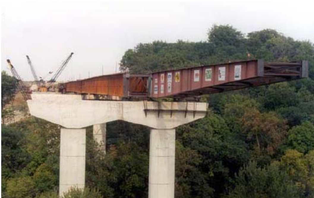
Figure 3.1. Horizontal launching of the Iowa River bridge, 92 meters long [4]
