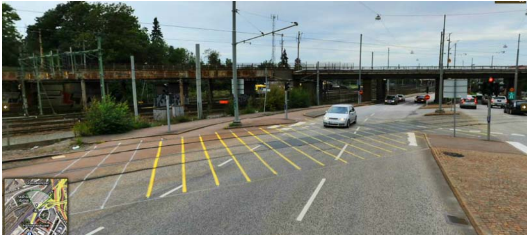
Figure 4.10. Street view of the Persontägsviadukten bridges (Source: Eniro)
