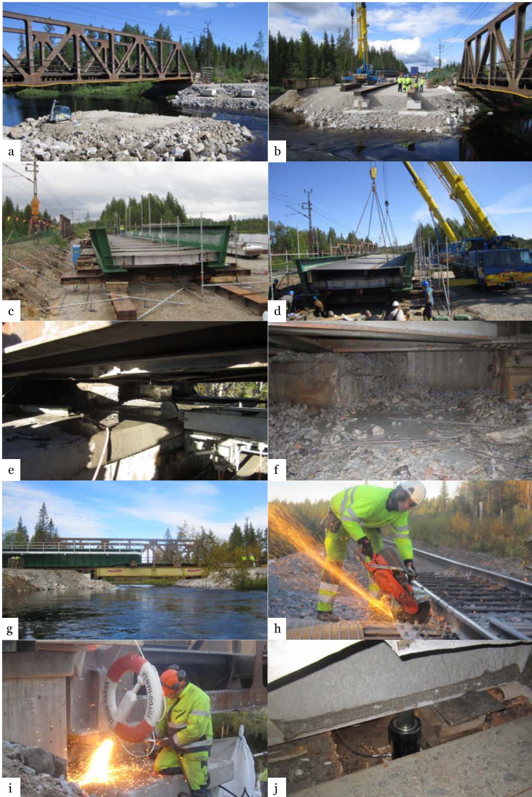
Figure 4.5. Building steps a-j for the replacement of the bridge over the Åby River [18]
