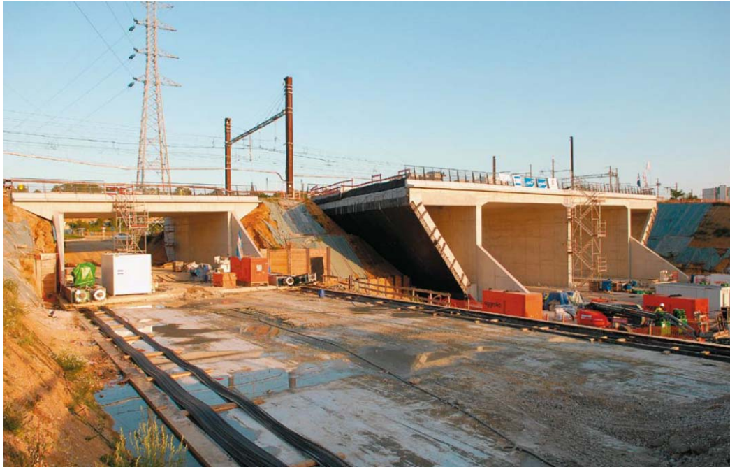
Figure 3.3. Installation of two bridges in Boissy-Saint-Léger, France by the techniques of Autofonçage® (left) and Autoripage® (right) (Source: Freyssinet)
