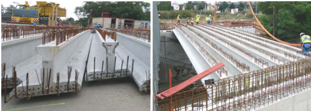
Figure 2.3. Installation of I-beams in UHPFRC at the Pinel Bridge (Source: Setra)
