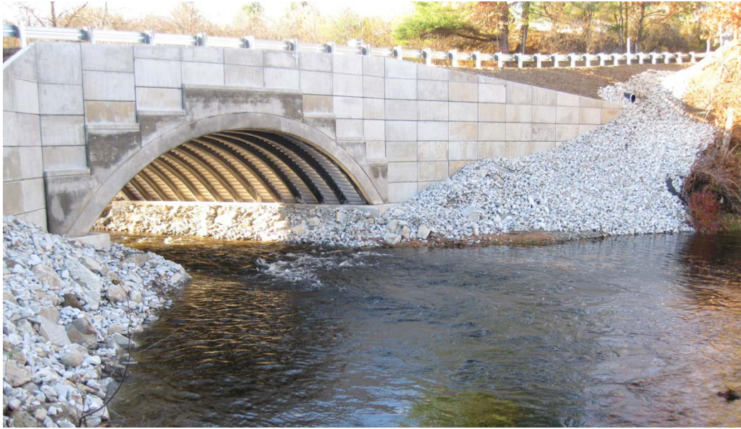
Figure 2.6. Bridge-in-a-Backpack built over the Royal River in Maine, USA (Source: Innovative Products)
