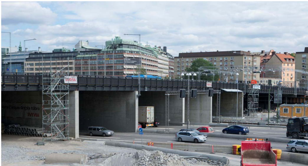
Figure 2.8. Temporary bridge with stress-laminated timber deck in Solna, Sweden (Source: Lennart Johansson, Stadsbyggnadskontoret, Stockholms stad)
