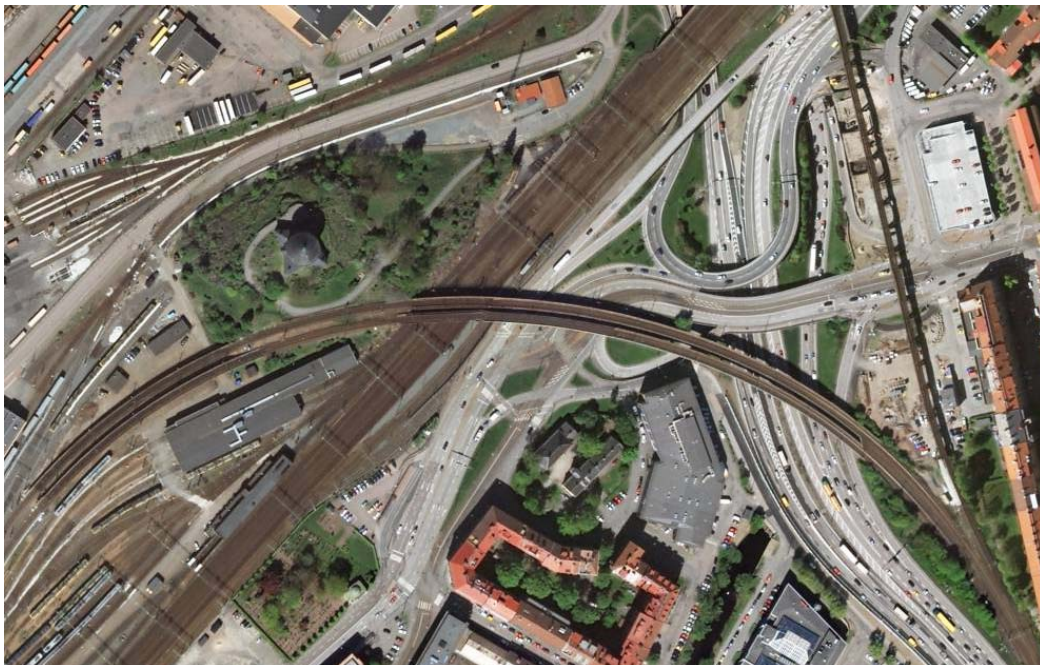
Figure 4.9. Aerial view of the Persontågsviadukten bridges (Source: Eniro)
