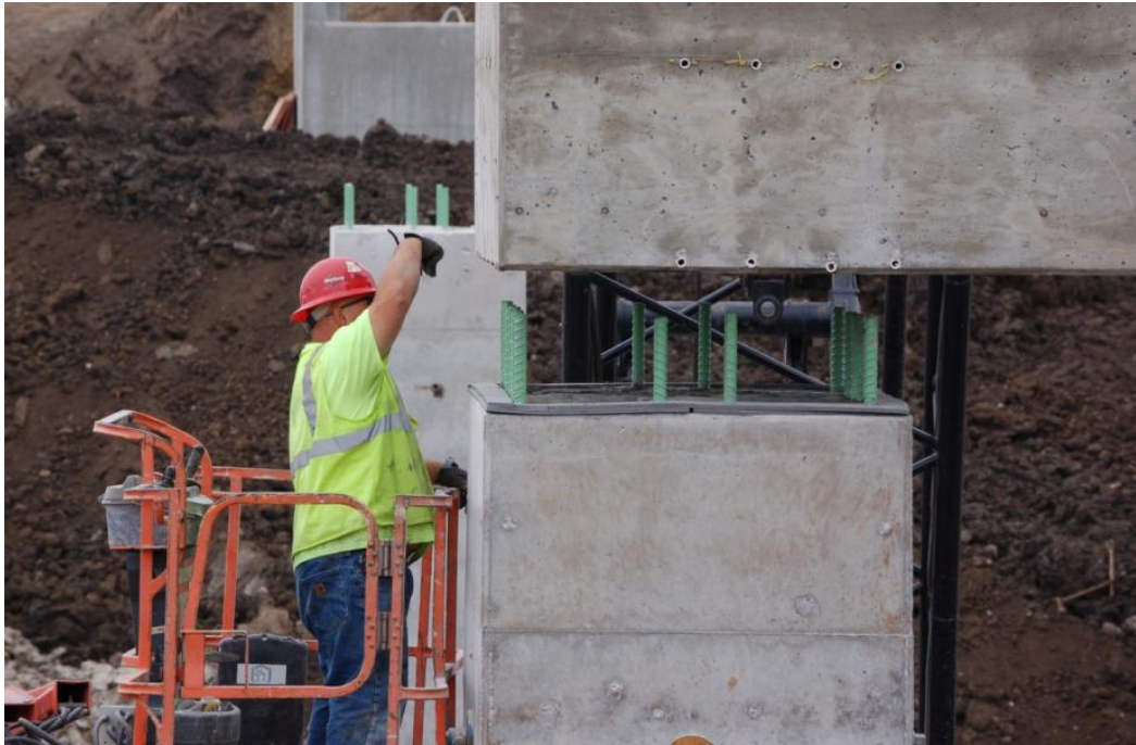
Figure 2.16. Installation of pier cap with grouted sleeve reinforcing bar couplers for the Bridge over Keg creek, Iowa, USA [Source: AASHTO]
