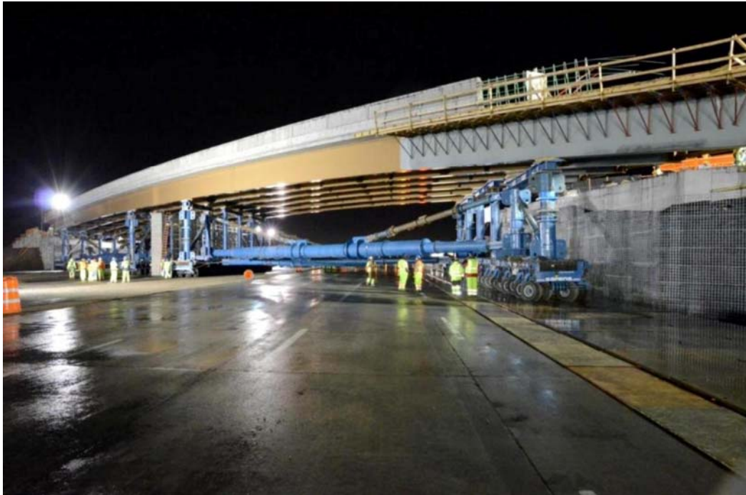
Figure 3.7. Installation of Sam White Bridge using SPMTs in Salt Lake City, Utah, USA (Source: Sarens)
