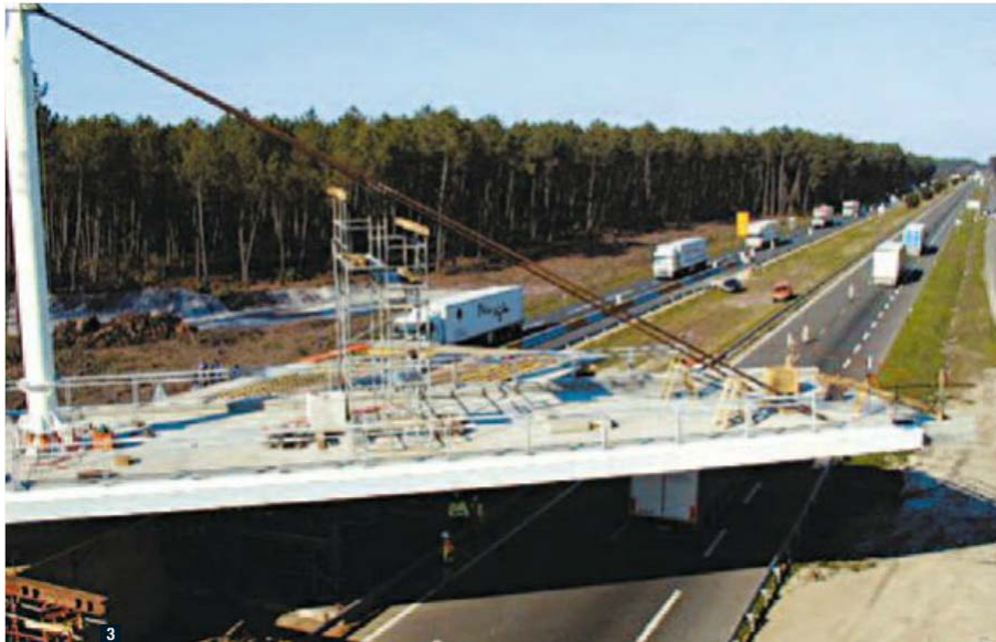
Figure 3.6. Installation by rotation of one the 11 bridges over RN10, France [5]
