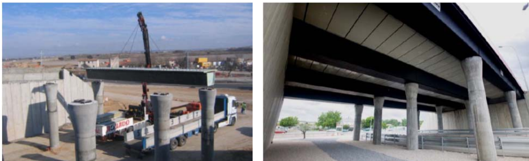
Figure 2.4. Installation of FRP girder at one of the M-111 bridges (left) and view of the completed bridge (right) (Source: Acciona)
