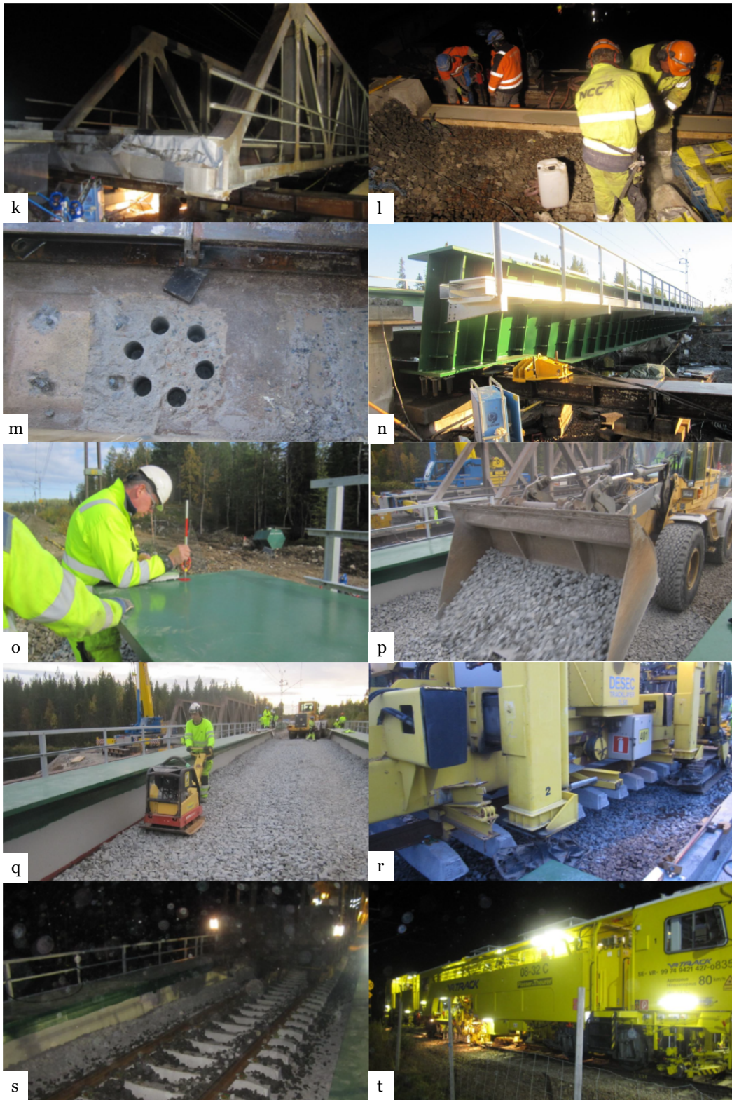
Figure 4.6. Building steps k-t for the replacement of the bridge over the Åby River [18]
